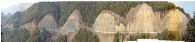
Figure 4. 11 slopes in the study subject area
