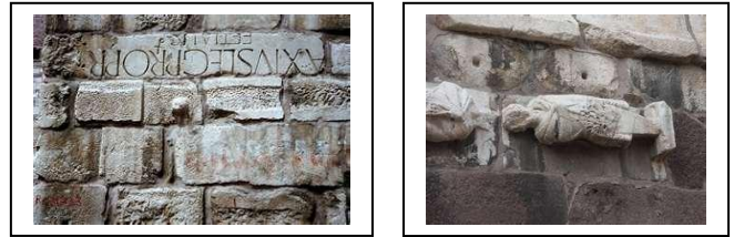
Plates 1 and 2: Examples of the Reuse of building Materials in the Citadel Walls, Ankara, Turkey
