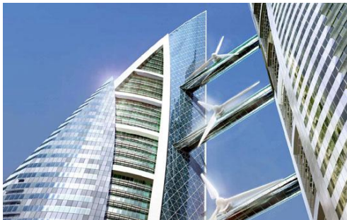
Figure 11: Bahrain World Trade Centre with Wind Turbines
