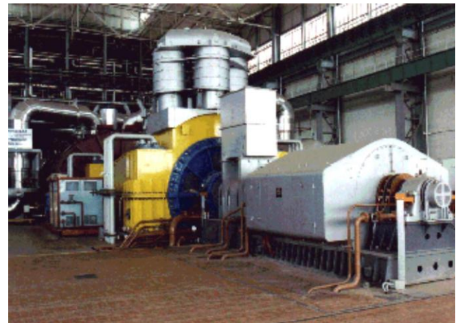
Fig. 4 – Side view on the TA from the side of the exciter. Connection between sensors INVA to HYNI
