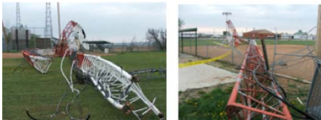
Figure 2.Examples of tower failure [5].
