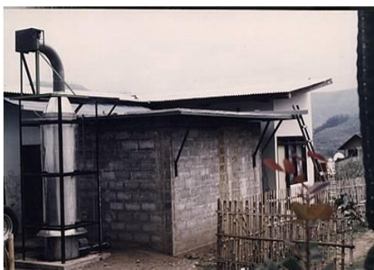
Figure 4. Hybrid nocturnal cooling for temporary cool storage in the highland of Malang, East Java[5].
