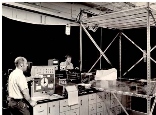
Figure 1. Rainfall simulator. Author at control panel, and Graduate Student James Cronn.
