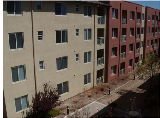
Figure 6: La Aldea Building Showing the Unshaded South Facade
